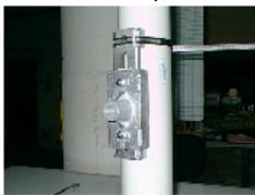
Wrap the first steel band around back plate at top and tighten down. Remove duct tape and place rod plate over stove bolts.
