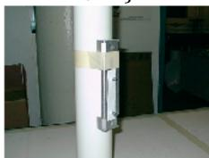
Place bracket plate at desired height on light pole and duct tape to pole to hold in place.
