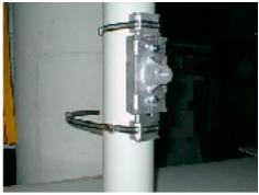
Install 2nd banding strap on bottom of back plate and tighten down.
